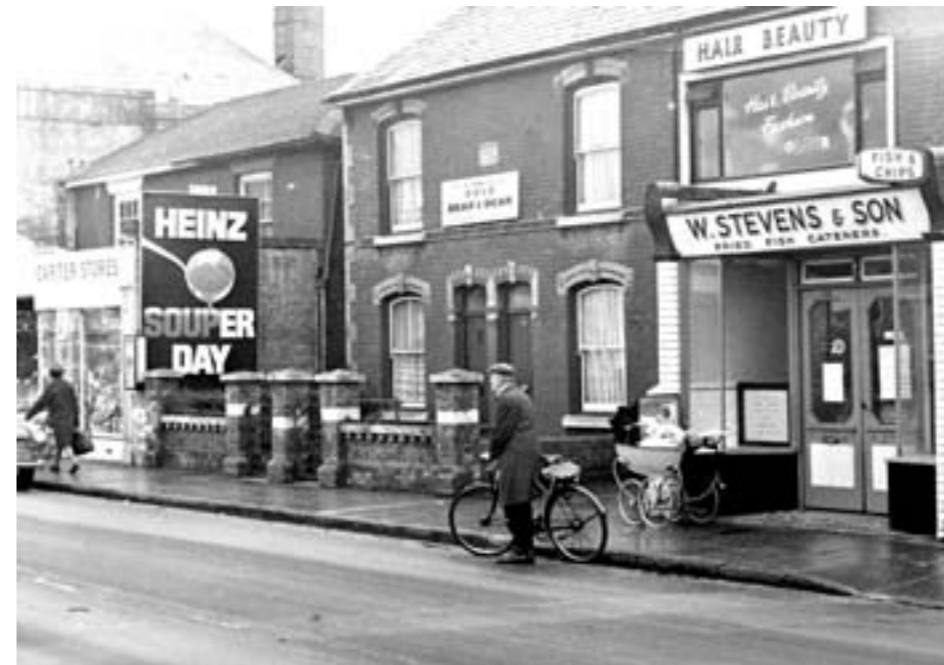
Stevens Fish and Chip shop on last day before demolition - Saturday 7th December 1968
