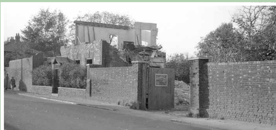
Demolition of Turret House, September 1956
