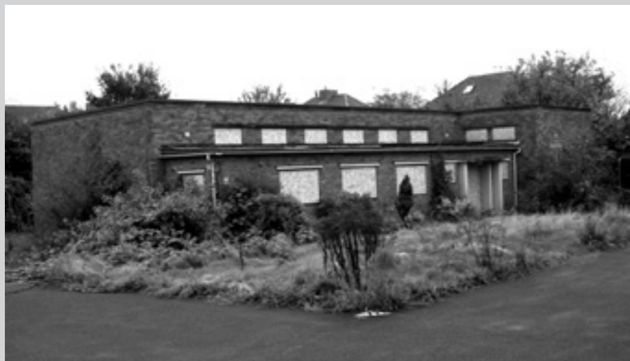
Former Catholic Church
